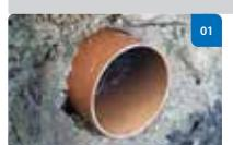
Clean the internal surface of the pipe from slurry and debris.
